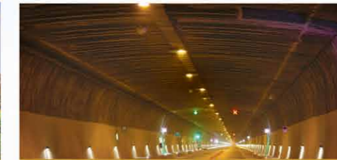
2017 Chenani - Nashri Tunnel, Jammu & Kashmir
