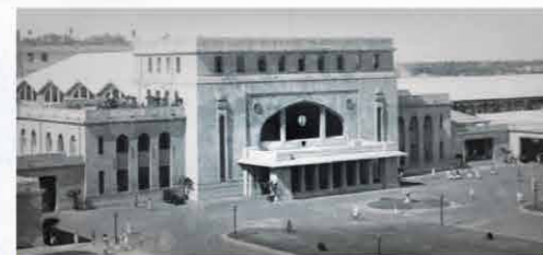
1930 Mumbai Central Station
